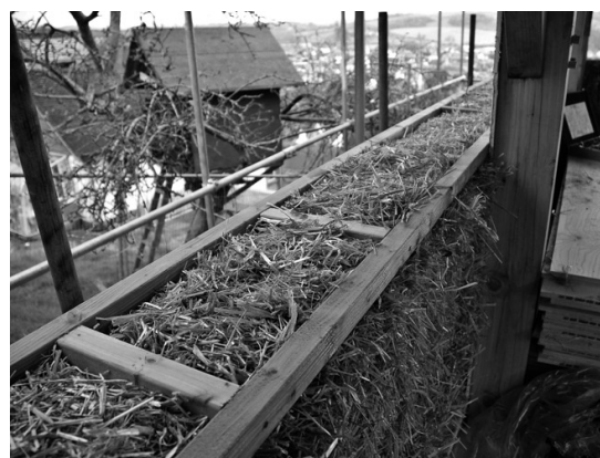
Figure 5: Timber ladder laid on every second course of bales
